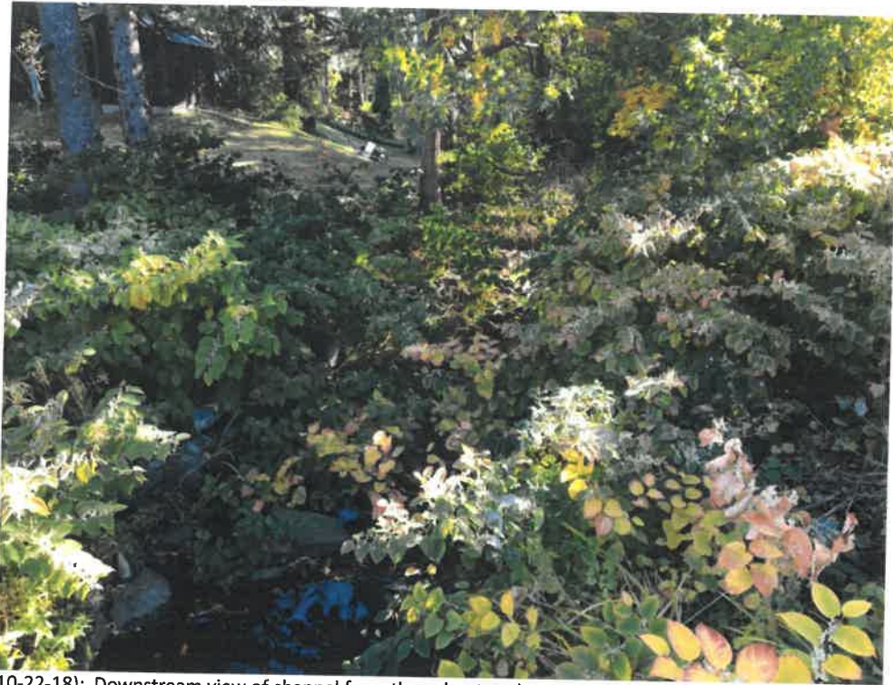
Photo 9 (10-22-18): Downstream view of channel from the culvert outlet rip rap plunge pool apron area on the east side of Shore Road. This flow travels to Casco Bay through the Delano Park neighborhood which is susceptible to high flow conditions.
