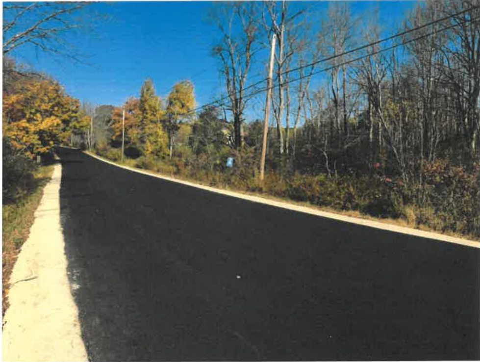
Photo 1 (10-22-18): Facing north at Eastman Road crossing of Trout Brook. Blue sign indicates that the culvert is within the Trout Brook Watershed which is an Urban Impaired Stream. Road freshly paved with new gravel shoulders.
