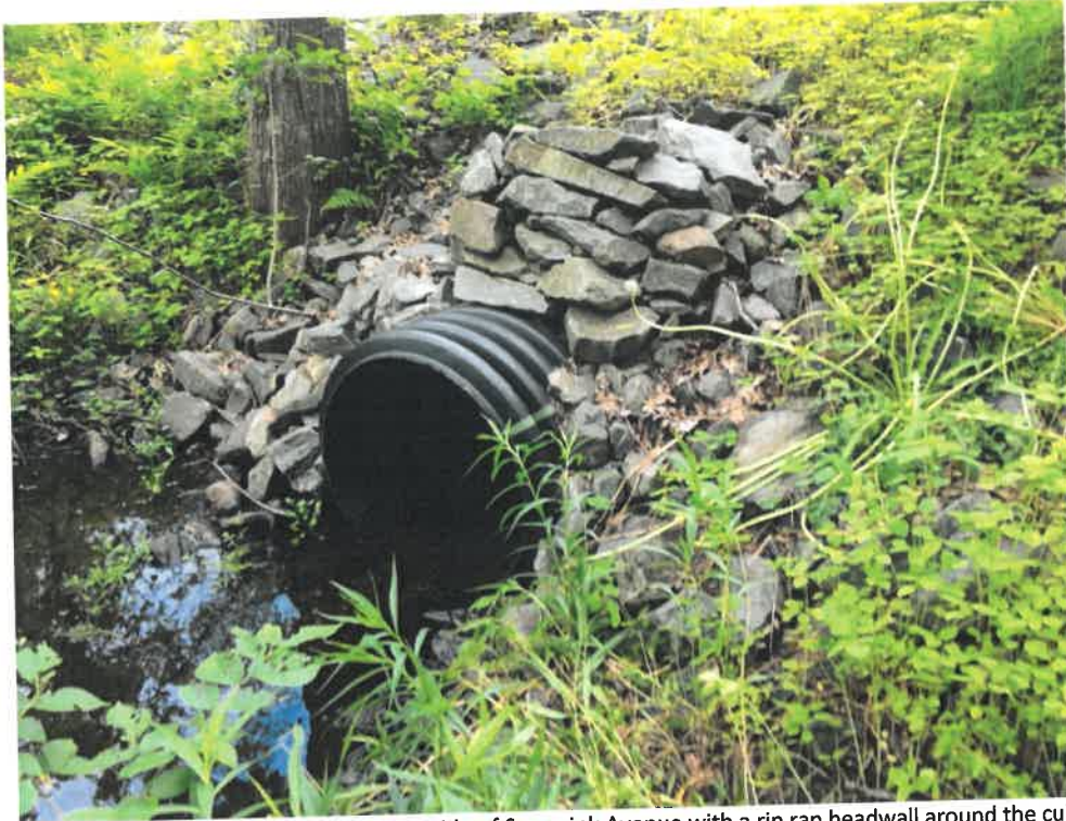
Photo 5 (06-06-18): Culvert outlet on west side of Spurwink Avenue with a rip rap headwall around the culvert.
