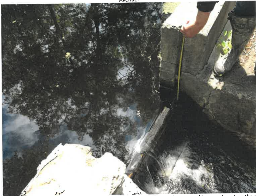
Photo 4 (06-06-18): Closeup view of adjustable elevation wooden board weir outlet to pond impoundment on the south side of Spurwink Avenue.
