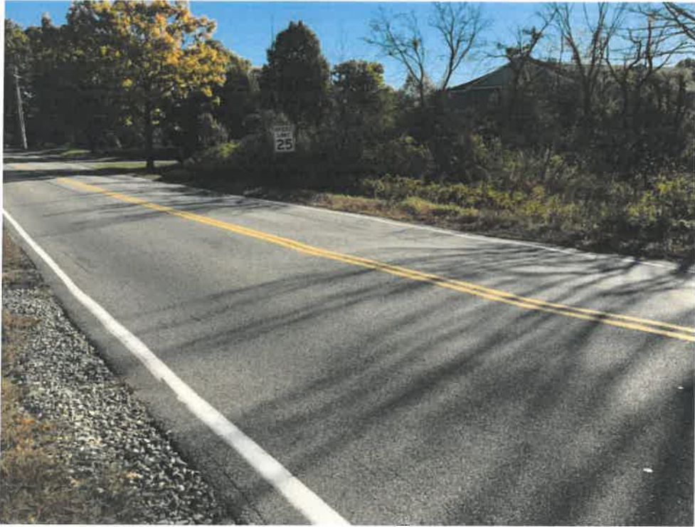
Photo 1 (10-22-18): Facing east at Scott Dyer Road at the Willow Brook culverts crossing.
