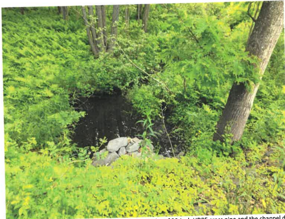
Photo 5 (06-06-18): Culvert outlet on west side of Spurwink Avenue with a rip rap headwall around the culvert.
