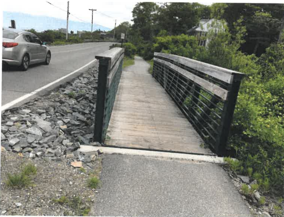
Photo 2 (06-06-18): Facing south at the Shore Road Path footbridge directly adjacent to the inlets of the three cross culverts.
