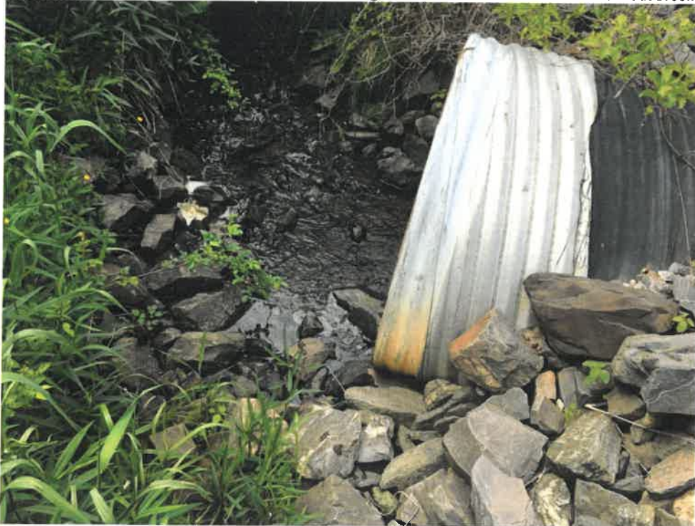
Photo 2 (06-06-18): Inlet of 60-inches wide by 44-inches tall corrugated aluminum elliptical cross pipe with rip rap apron and headwall. Flow curls into culvert abruptly after flowing southerly along and parallel to Spurwink Avenue.
