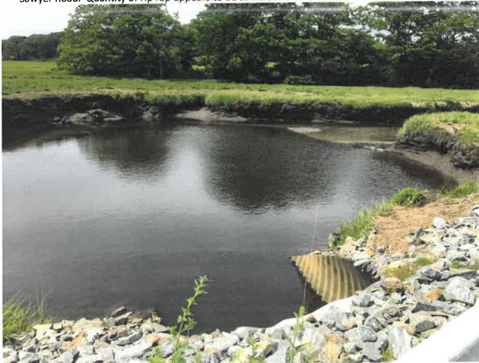
Photo 6 (06-06-18): Overhead view of culvert outlet and the widened area of the Spurwink River beyond the culvert outlet. The Spurwink River channel flows to the north (right hand side of this photo).
