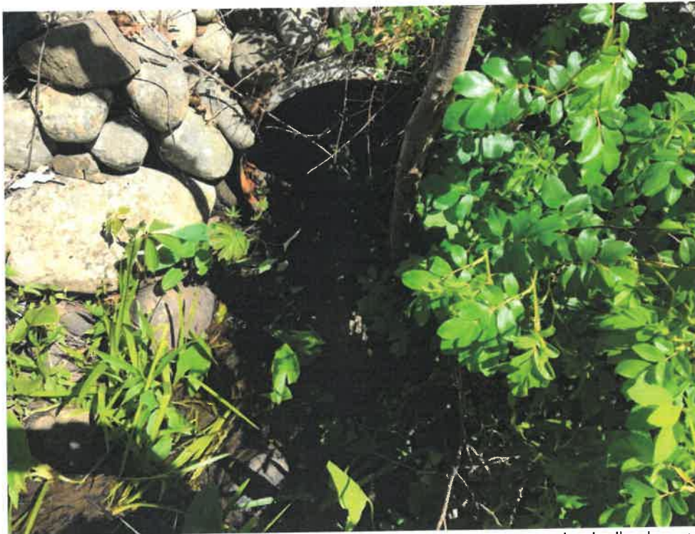
Photo 2 (06-06-18): Inlet of 24-inch corrugated aluminum cross pipe with a rip rap creating a headwall and apron. Inlet is on the west side of Spurwink Avenue and very thick vegetation made locating the culvert difficult.
