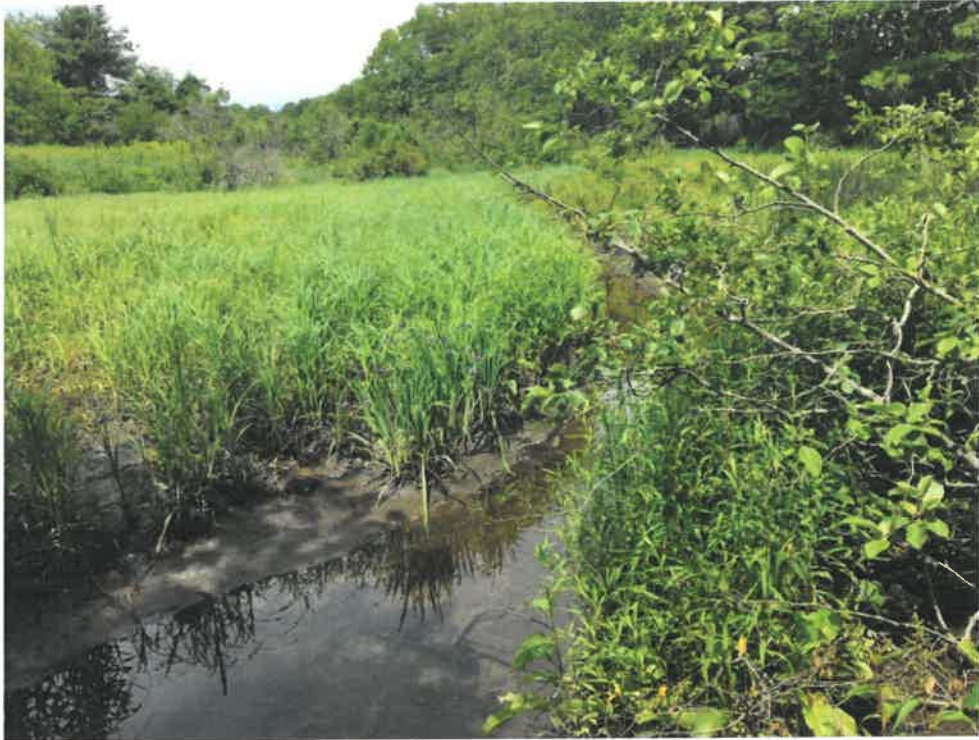
Photo 5 (06-20-18): Upstream Willow Brook channel flows southerly through a wetland area to reach culvert.
