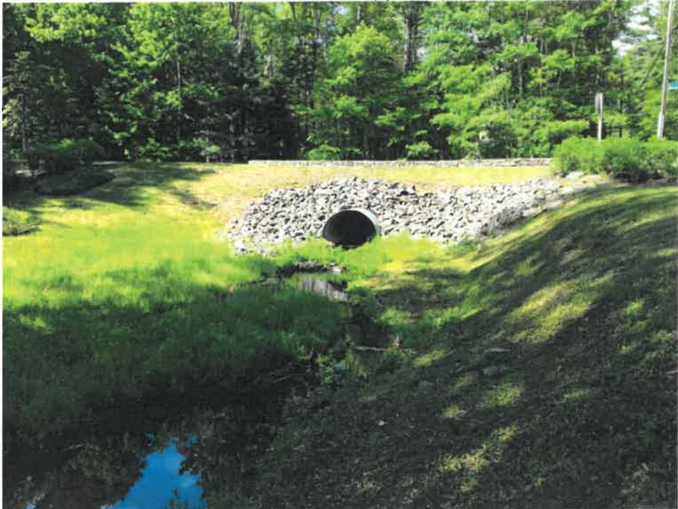
Photo 4 (06-06-18): Facing northwest from the Mitchell Road culvert toward the 3-feet tall by 4-feet wide elliptical culvert under nearby Hobstone Road with channel of the Pond Cove Brook upstream of the Mitchell Road culvert inlet.
