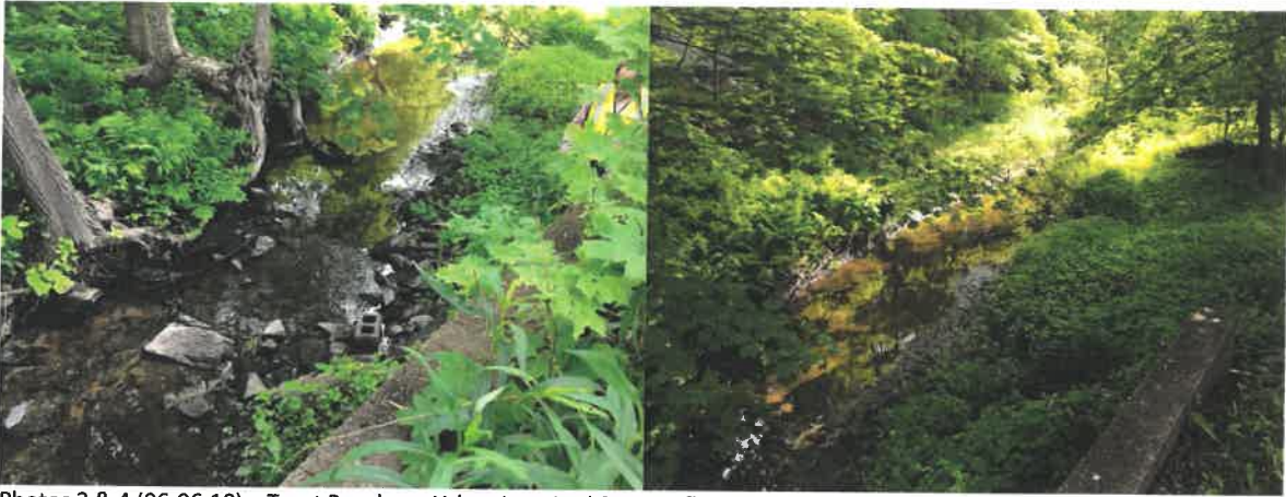
Photos 3 & 4 (06-06-18): Trout Brook, an Urban Impaired Stream, flowing to the culvert inlet on east side of Route 77. Photo 3 is taken adjacent to the inlet and shows eroded areas at the base of the mature trees lining the northern bank. Photo 4 depicts a more uniform and stable channel further upstream from the culvert inlet.
