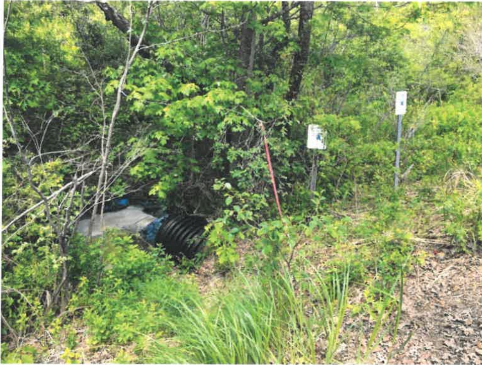
Photo 7 (06-06-18): Looking north down the Spurwink Avenue embankment at the outlet of the 36-inch HDPE culvert on the north side of Spurwink Avenue. Signs indicate the presence of the National Wildlife Preserve with the pink flagging tied to a survey pin.
