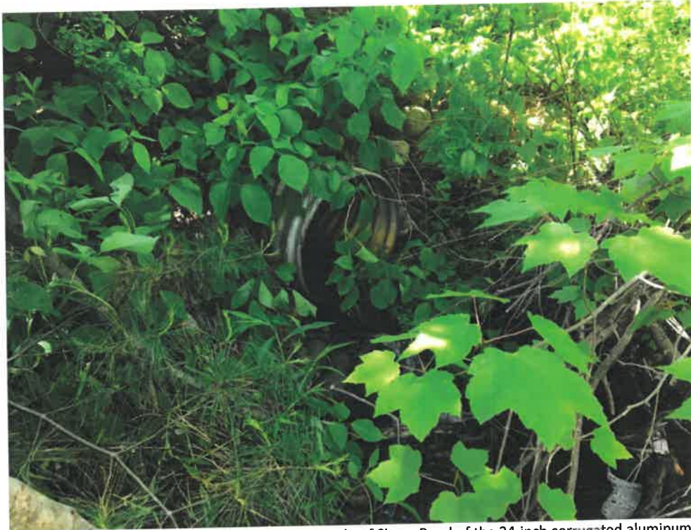
Photos 3 (06-06-18): Hanging culvert outlet on east side of Shore Road of the 24-inch corrugated aluminum pipe.
