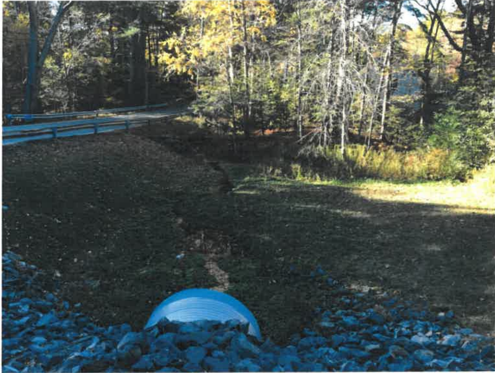
Photo 5 (10-22-18): Facing southwest at discharge flow channel of Pond Cove Brook from elliptical culvert under Hobstone Road to the Mitchell Road culvert inlet.
