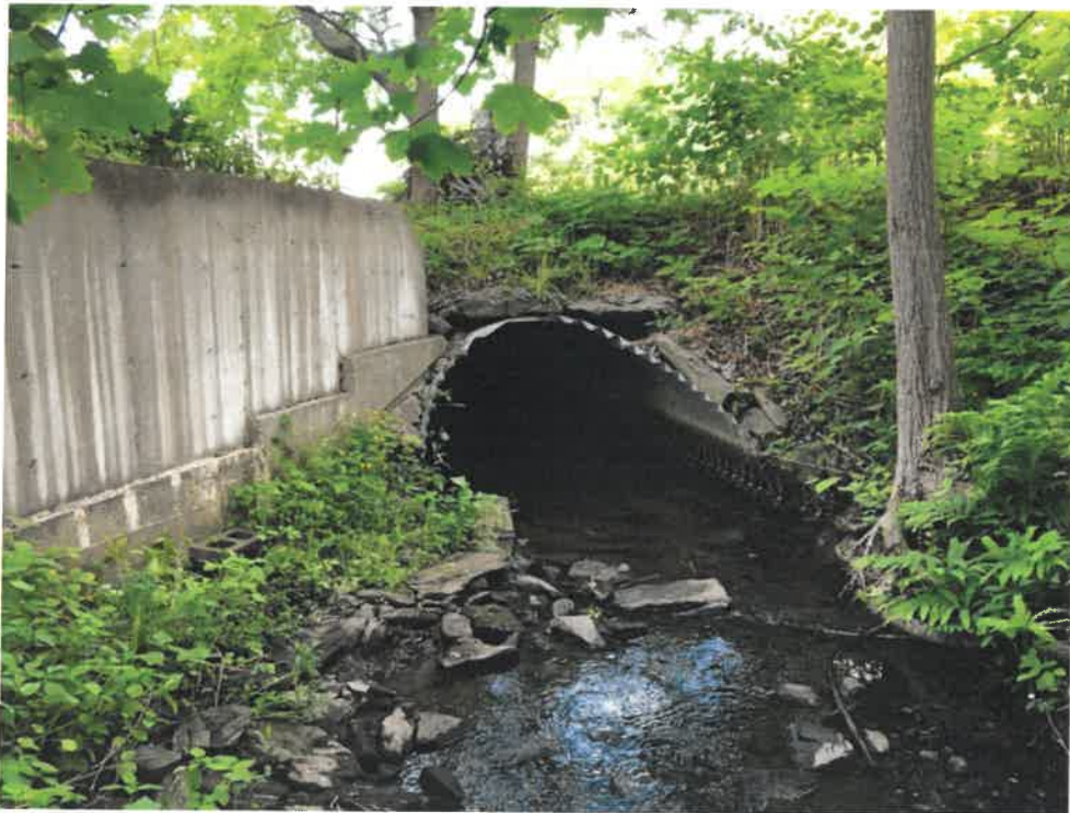
Photo 2 (06-06-18): Looking at the submerged Inlet of 8 foot, 2-inch-wide by 5 foot, 9-inch-high steel plate pipe arch cross pipe with concrete wingwall on the south side of Trout Brook. Inlet is on east side of Route 77.
