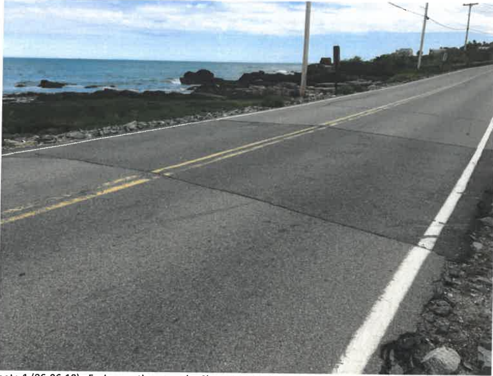
Photo 1 (06-06-18): Facing southeast at the Shore Road culvert crossing with Pond Cove in the background.
