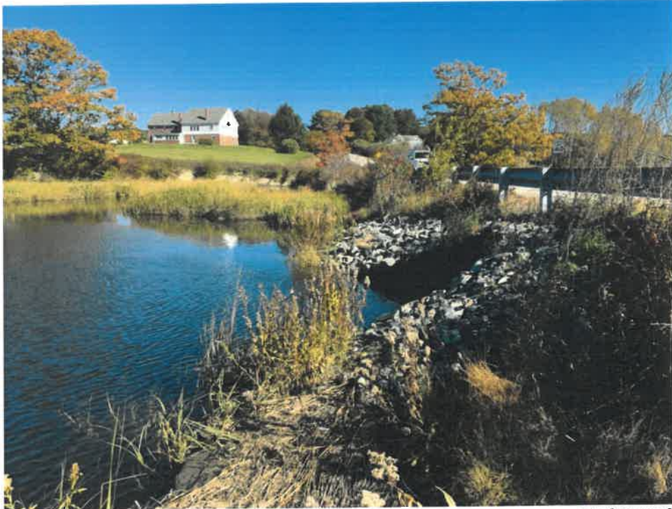
Photo 7 (10-22-18): Facing north during high tide of the Spurwink River on the outlet to the west of Sawyer Road.
