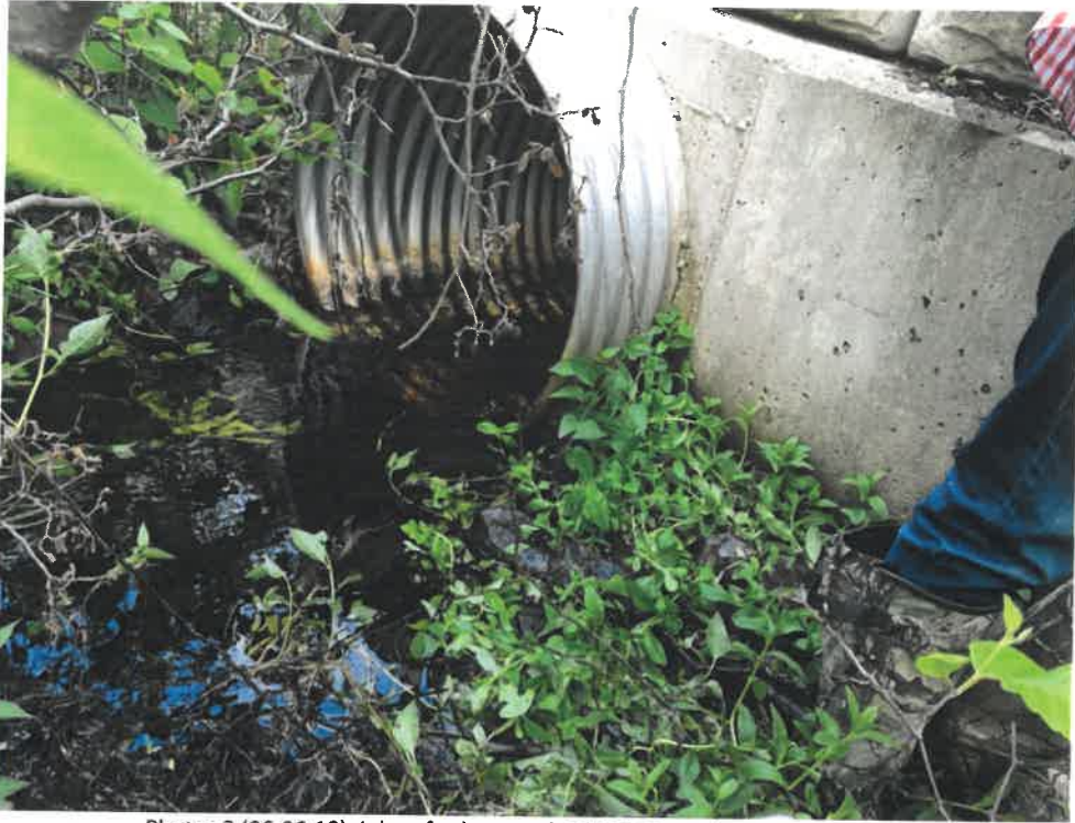
Photos 3 (06-06-18): Inlet of submerged culvert on west side of Shore Road.
