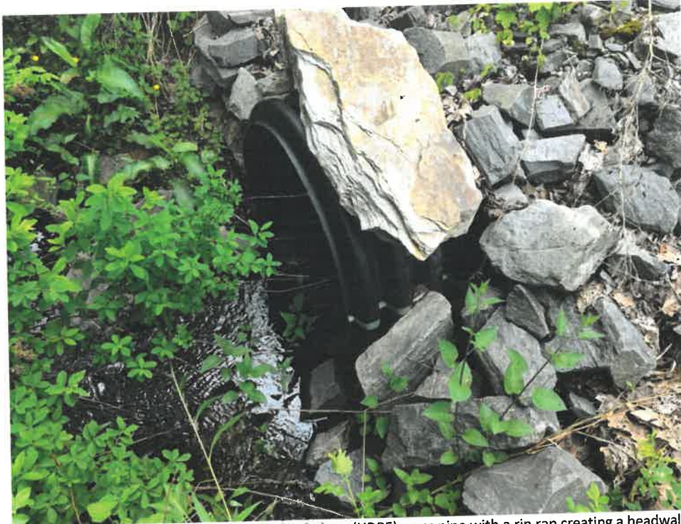
Photo 3 (06-06-18): Inlet of 30-inch High Density Polyethylene (HDPE) cross pipe with a rip rap creating a headwall and apron. Inlet is on the east side of Spurwink Avenue. Access to the culvert and the area around the inlet is relatively clear of vegetation.
