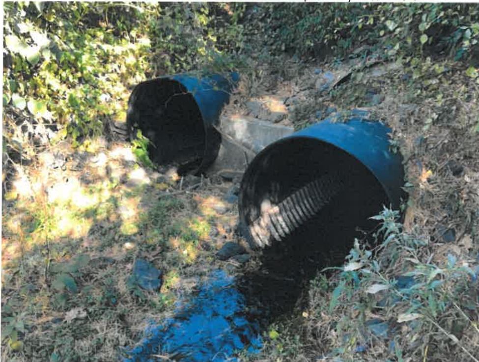
Photo 2 (10-22-18): Inlet of two 48-inch high density polyethylene liner pipes within the original corrugated aluminum cross pipes. Southerly culvert on the right-hand side conveys main flow of Alewife Brook with left-hand side culvert available for overflow capacity.
