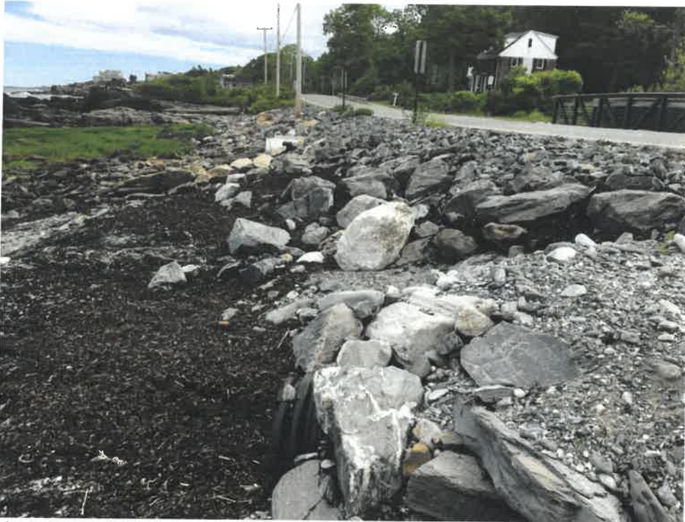
Photo 5 (06-06-18): Facing south along the rip rap armor of the oceanside outlet (west) side of Shore Road with Aluminum corrugated pipe outlet visible within the rock slope in the center of the photo.
