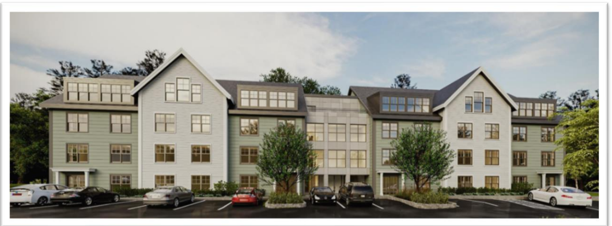
Figure 2: Dunham Court Multiplex building as seen in “Proposal for Housing at Ocean House Commons” presented by The Szanton Company.
