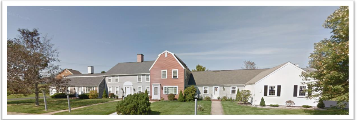
Figure 1: Colonial Village Condominium as seen on Starboard Drive in Cape Elizabeth.
