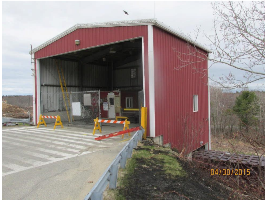
Photo #1 – Exterior view of west (front) and south (side) elevations.
