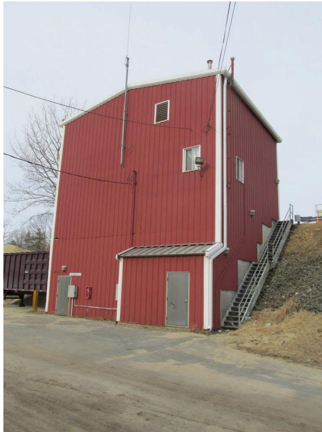
Photo #2 – Exterior view of east (back) and north (side) elevations.
